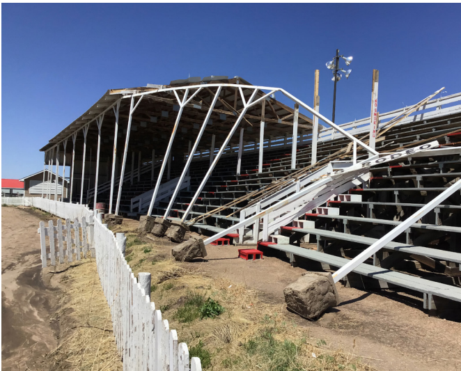
Top: Dust storm begins in North Platte. Left: The Grandstand at Nebraska's Big Rodeo in Burwell suffered damage as a result of the straight-line wind event in May 2022. Right: damage to the backside of the damaged grandstands.
