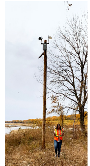
The Platte River Gauge project installed five river monitoring cameras and two river gauges along the Platte River to monitor river conditions. (Right) NEMA Program Specialist Marisa Alvares inspects the camera mounted at the top of a pole.
